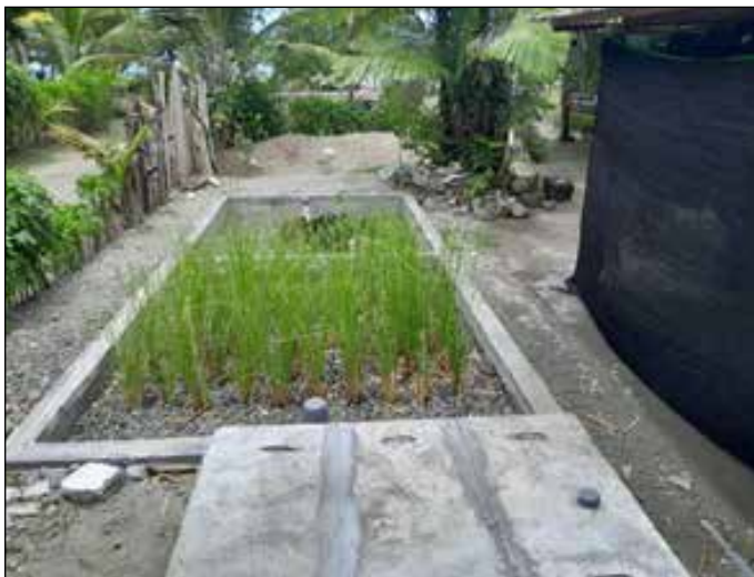
The finished constructed wetland systems with a septic tank followed by a gravel/rock constructed wetland followed by a small seepage bed.
