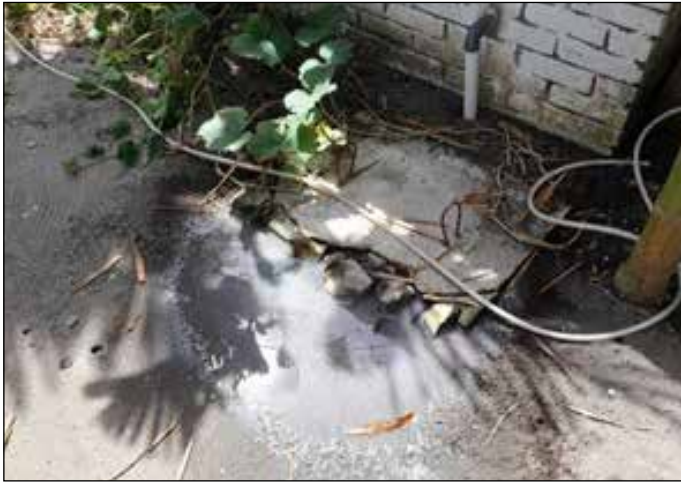
The before pictures show the surfacing wastewater from the systems that were eventually replaced with the constructed wetland systems above.
