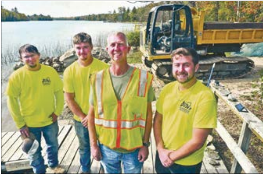
The Viita crew for this particular job included (from left) Charlie Lorfald, operator; Zach Cheney, operator; Rick Viita, owner; and Spencer Viita, estimator.
