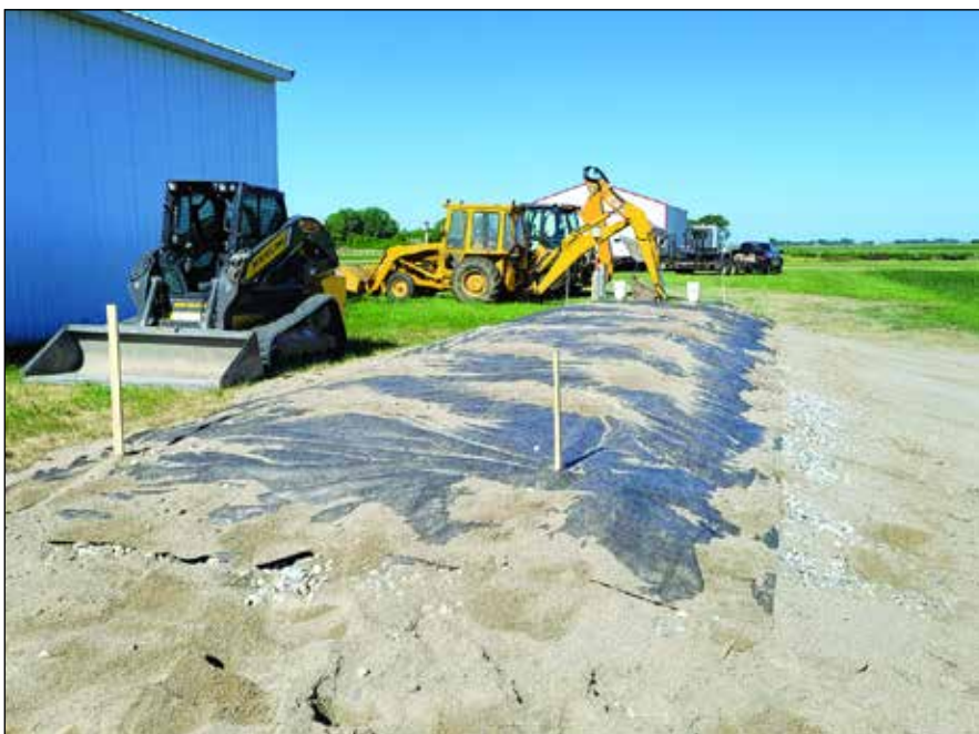
Part of documenting a job correctly is using photos. Capturing images is easy to do with phones these days and should include the entire installation from start to finish and even the equipment used.
